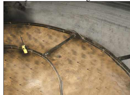
Typical installation arrangements of wall supports, brackets and circular supports at one of the site in Southern India. Location : Mangalore
