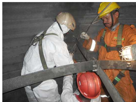
Bracket installation underway in a VGO reactor. Location : Bhatinda Client : HMEL. Licensor : Axens
